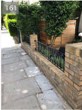
161 Half brick wall with metal trellis rail, in good condition.
