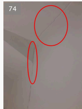
Crack separation on the wall to ceiling on 3 sides of the perimeter.
