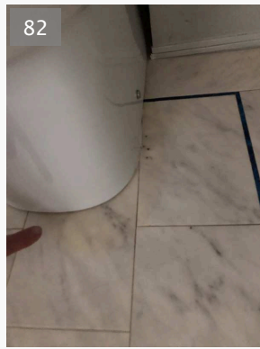
Leaking water closest. Note this aligns approximately with ceiling below. 24/02/2021 14:07 (GMT) at 51.57144640530343°, -0.1298319029032252°
