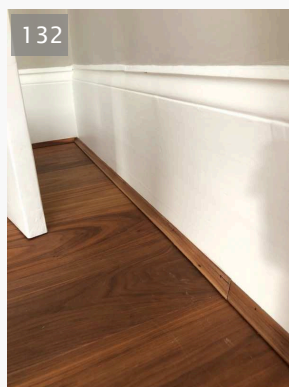
Baseboard generally in good condition. 24/02/2021 14:15 (GMT) at 51.57139650086744°, -0.1297354636375956°
