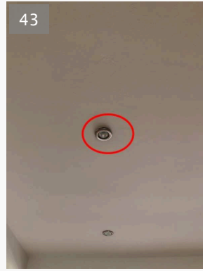
1 light fixture pulling out of the ceiling. All others are functional.
