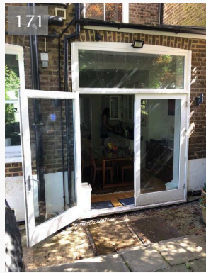
Rear wooden french doors, appears serviceable, useable condition. 24/02/2021 15:10 (GMT) at 51.57143990998938°, -0.1298172316053907°
