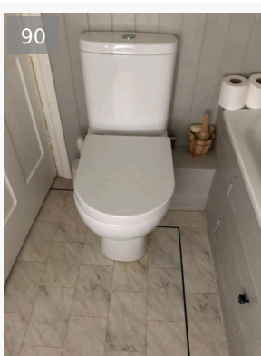
Toilet is leaking. Note stains on floors.
