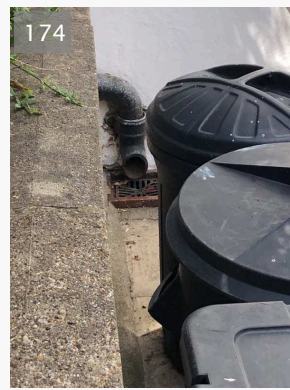
Downpipe termination at adjacent property to the right of subject property showing termination at catch basin. 24/02/2021 12:26 (GMT) at 51.5715256366576°, -0.1298390105448993°
